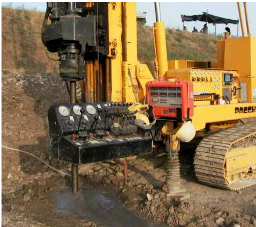
Fig. 6. Registration of data during Jet Grouting injection.
