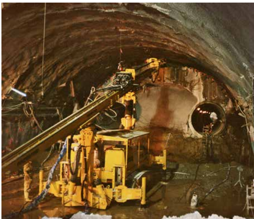
Fig. 6 - 7. View of the P 1500 TAF drill rig used for consolidation of the vault.
