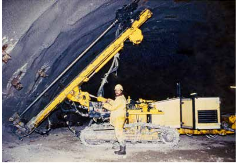
Fig. 9. PRP 105 D drill rig consolidating the piers.
