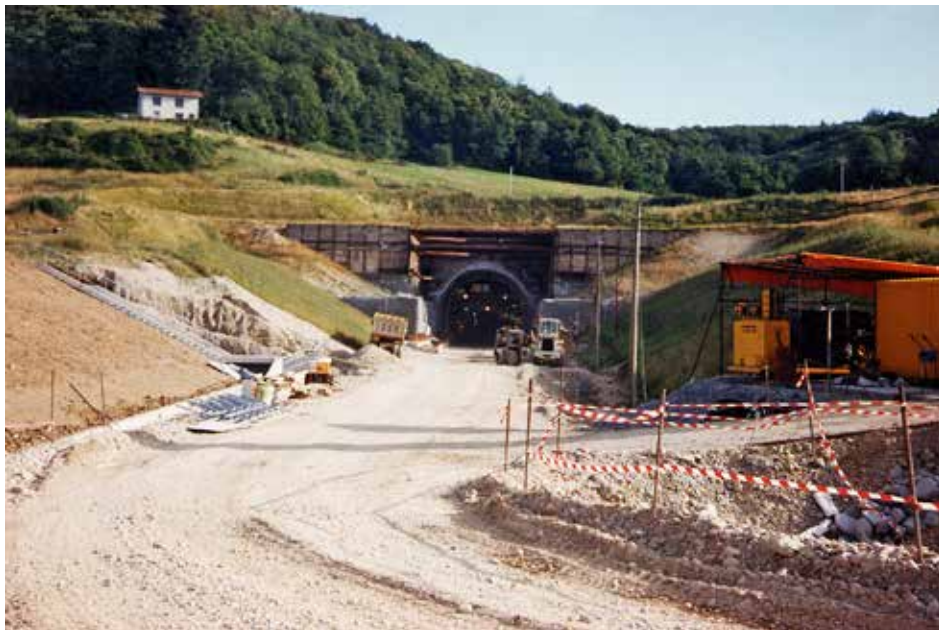
Fig. 1. View of tunnel entrance.
