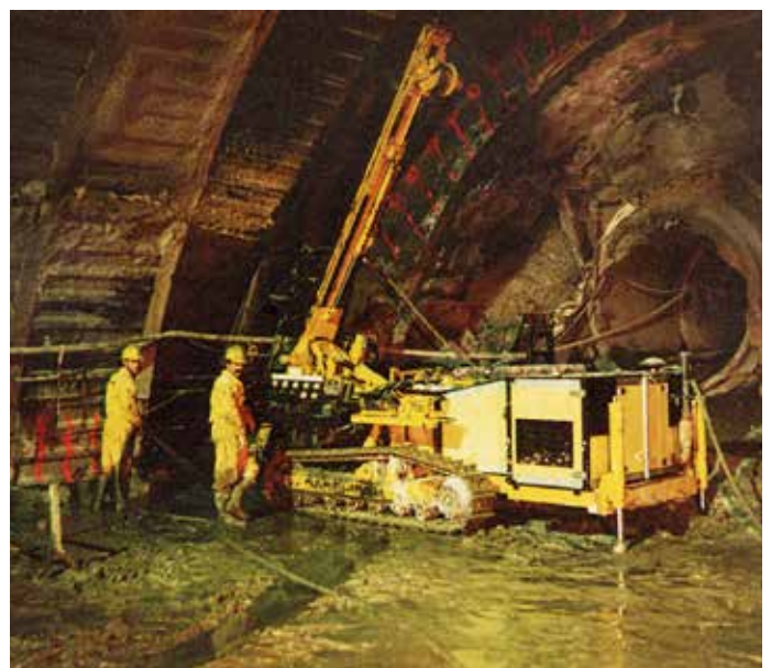
Fig. 11. PRP 105 D drill rig during construction of the reinforced columns.
