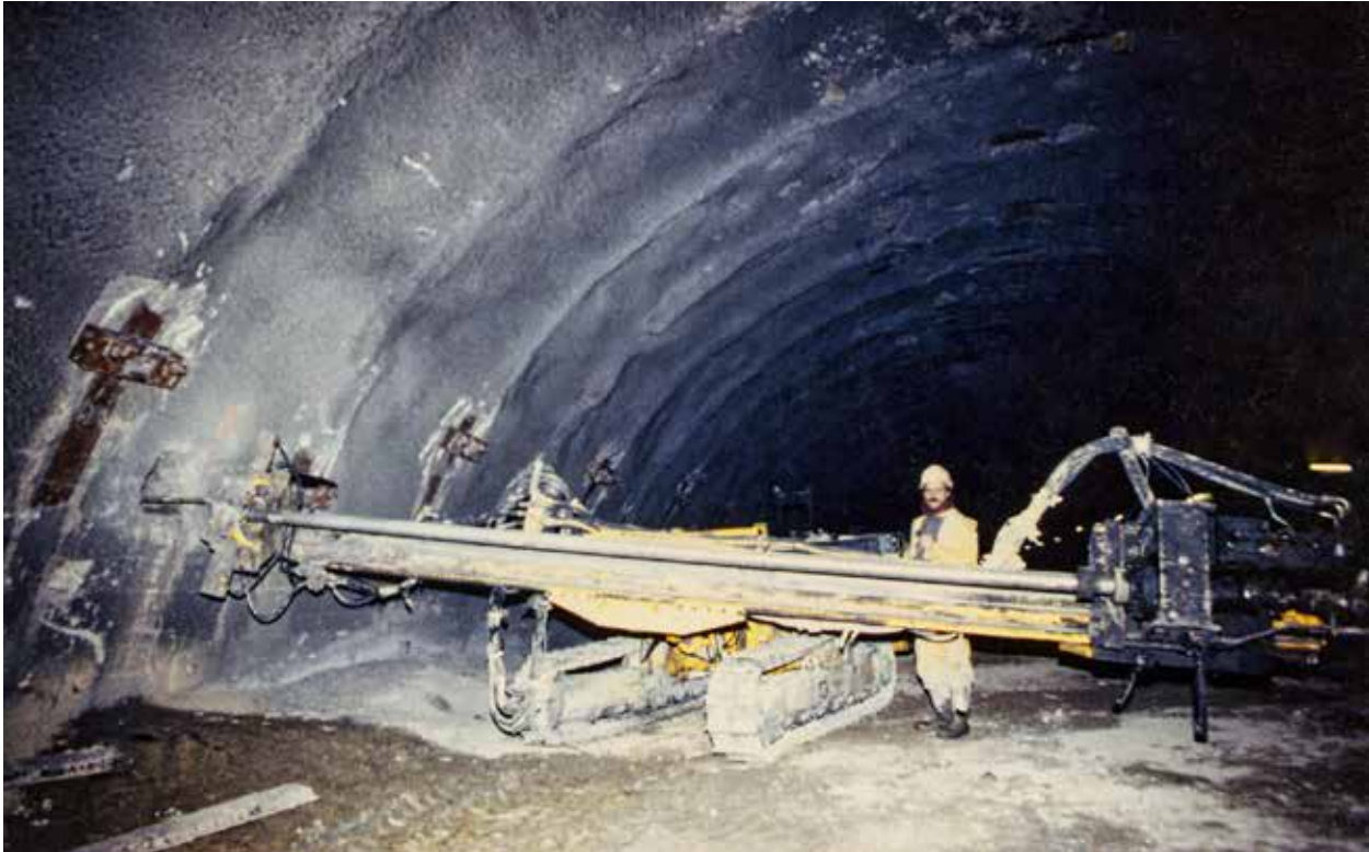
Fig. 12. PRP 105 D drill rig during anchorage of the cambers.
