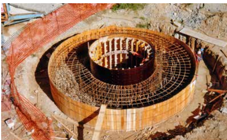
Fig. 8. Reinforcement of shaft bead.
