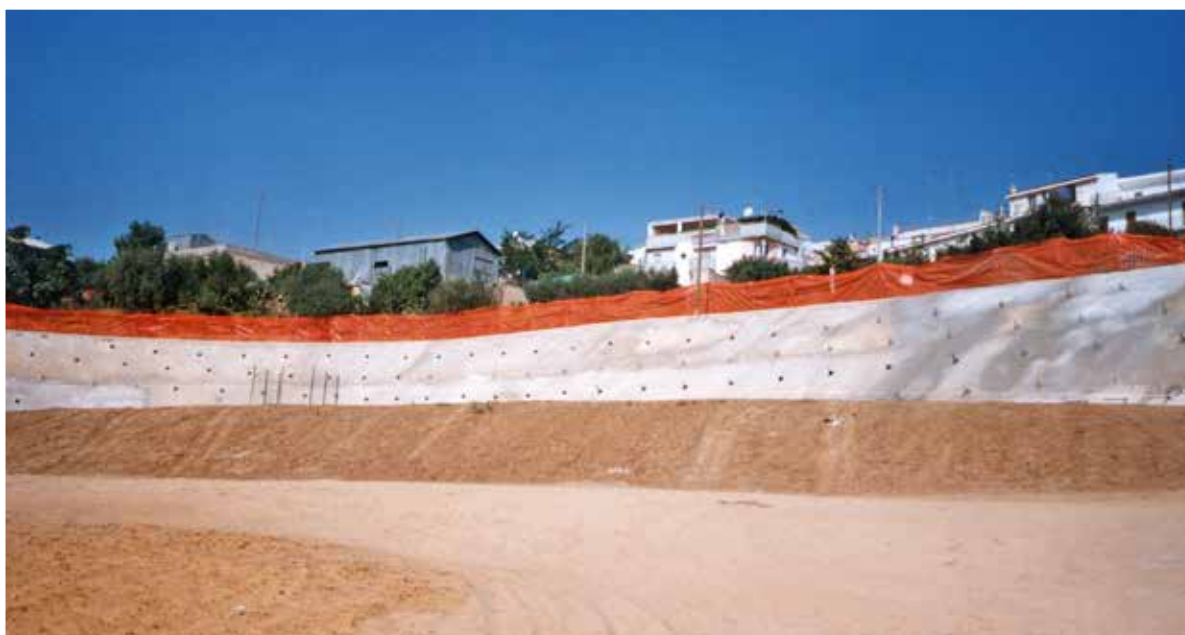
Fig. 1. Main nailed wall.
