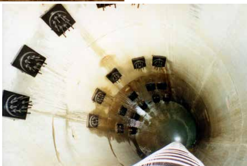
Fig. 10. Inside of shaft with a view of the tie rod heads.
