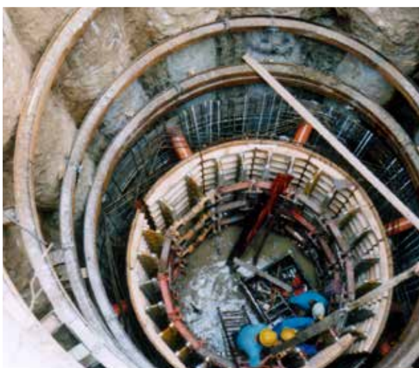
Fig. 6. Formworks assembly stage.
