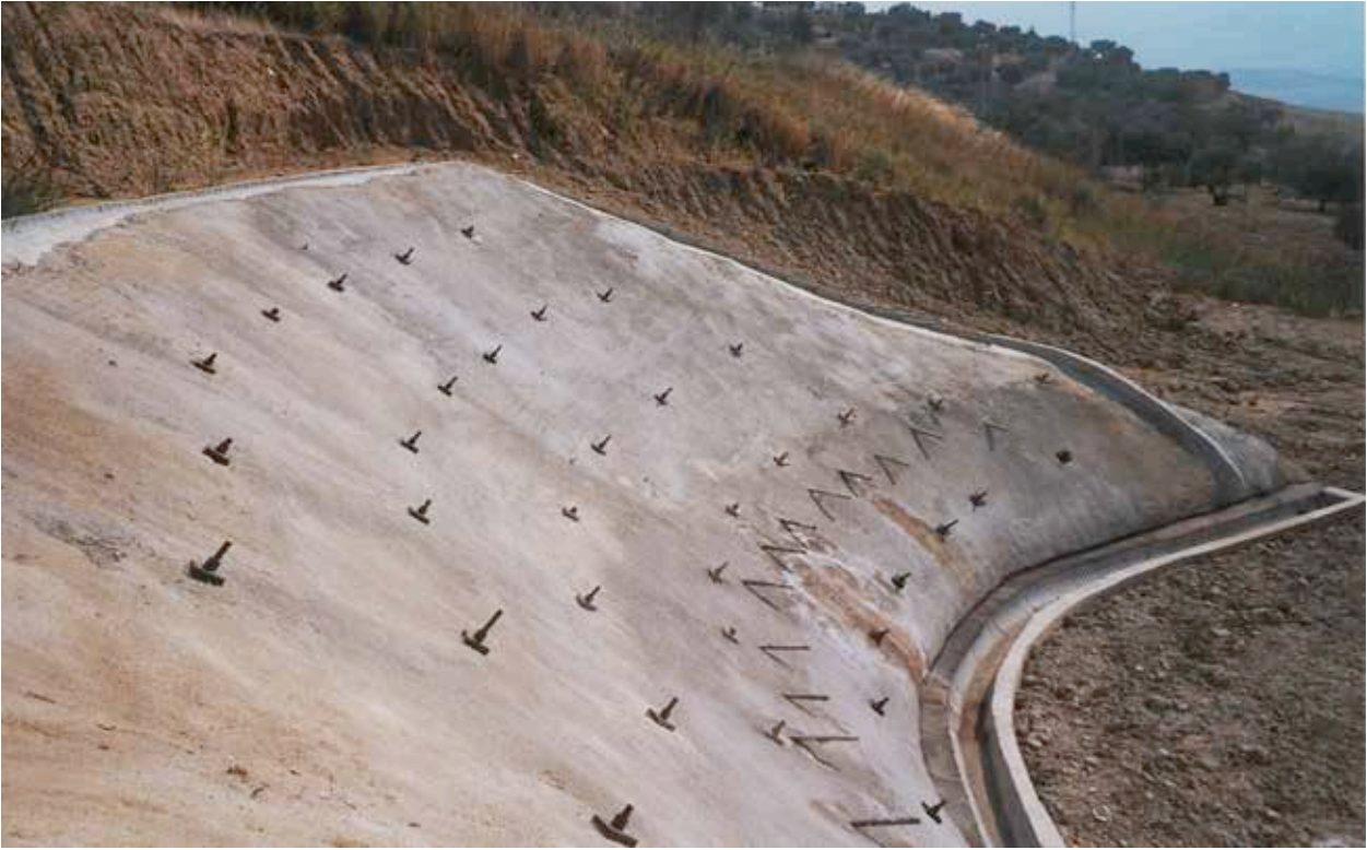
Fig. 12. View of the nailed wall.
