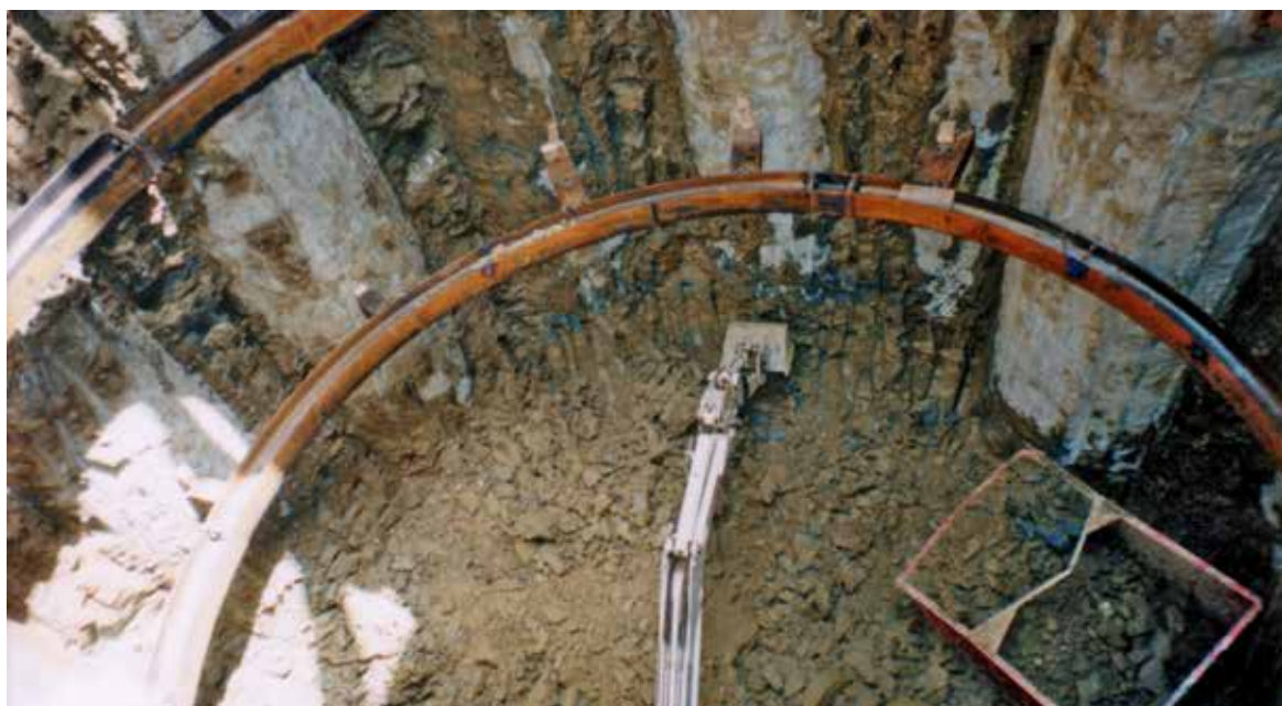
Fig. 5. Camtering installation stage.
