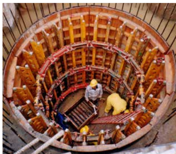
Fig. 7. Shaft lining stage.
