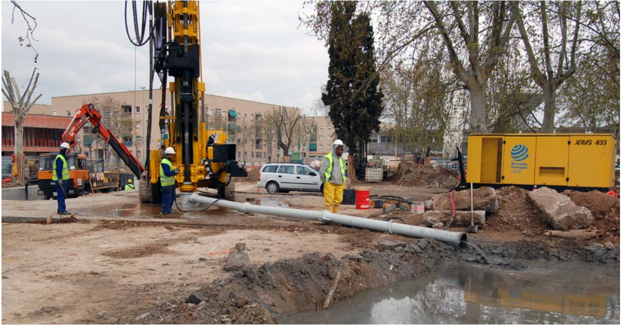
Fig. 31. Recovery of drilling/injection fluids and conveyance to decanting tank.
