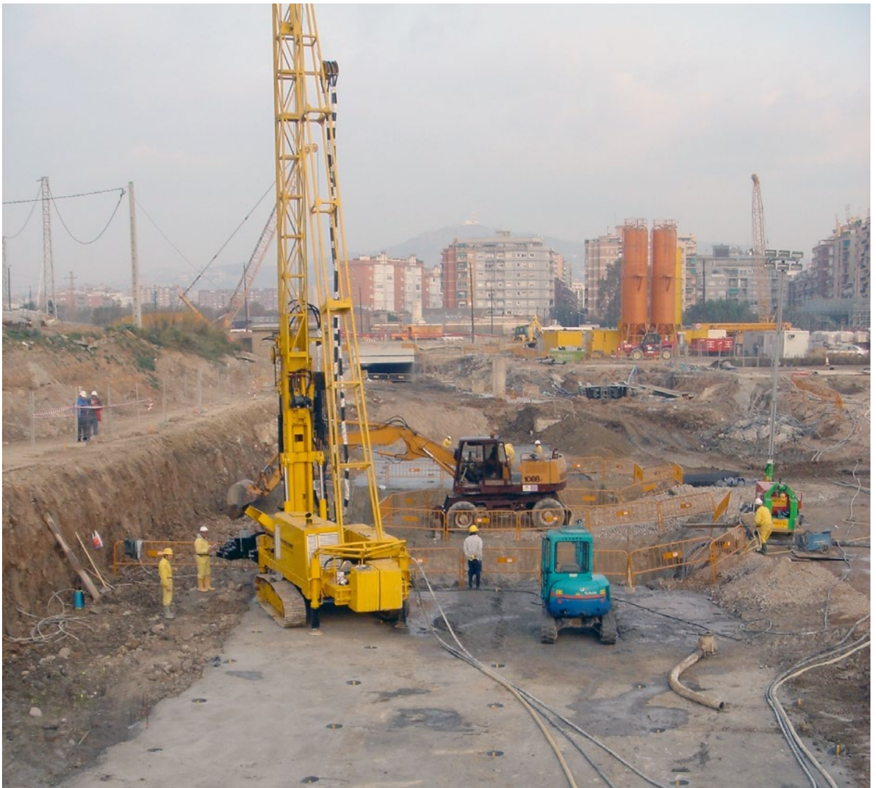
Fig. 32. PACCHIOSI P1500 hydraulic drill rig model ES with extension; work on the surface; the silos for storage, dispensing, mixing and pumping the cement mixtures are visible in the background.
