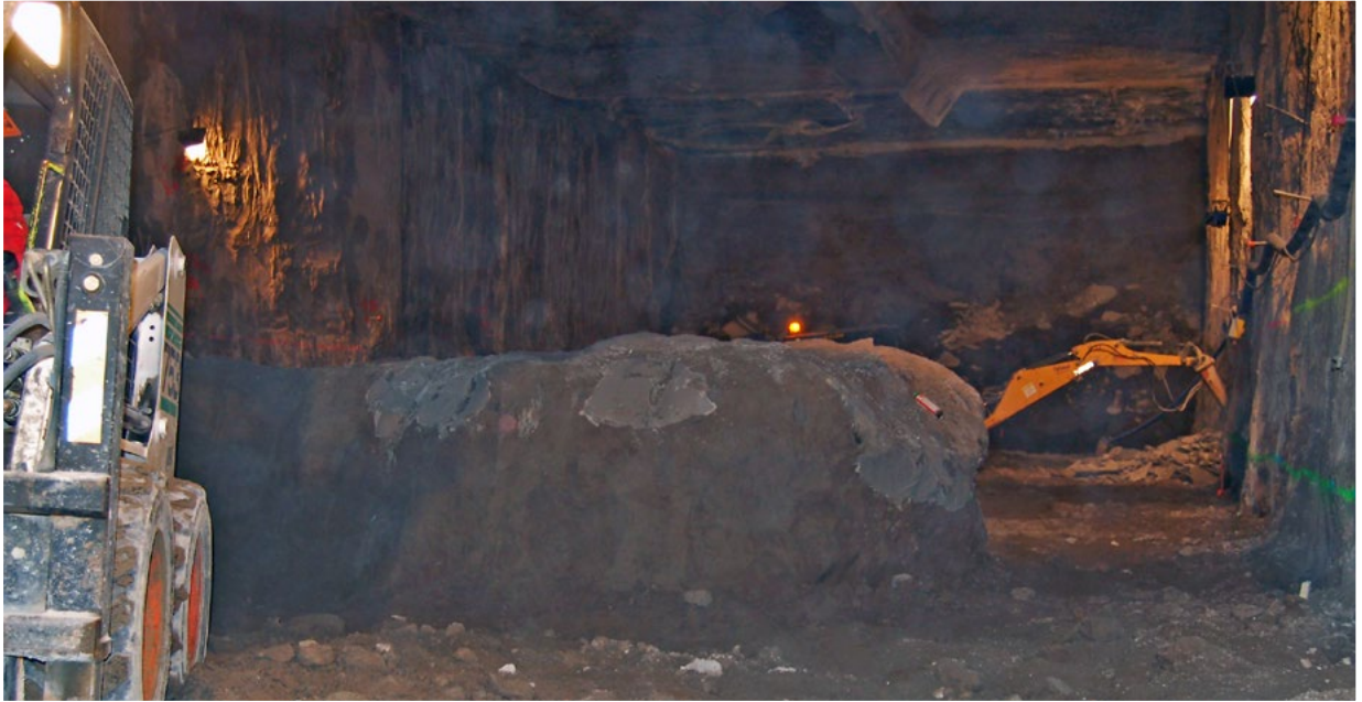
Fig. 18. Summit of an uncovered column measured directly: Ø over 4 m.
