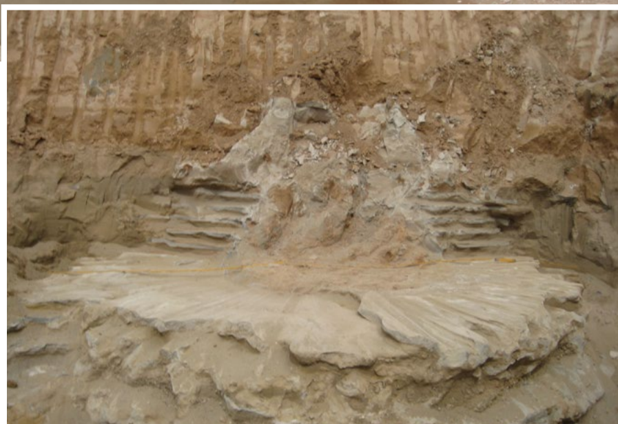
Fig. 23-24. Detail of uncovered column, diameter Ø over 5 m.
