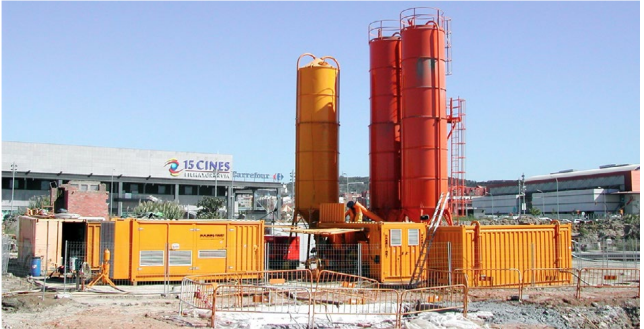
fig. 39. Fixed worksite installations; silos for storage of cement (2) and bentonite (1), dosing and mixing unit (PACCHIOSI MA 2000 mixer) and PACCHIOSI LASER pump mod.2800 for water and cement mixture; containers for workshop and warehouse.
