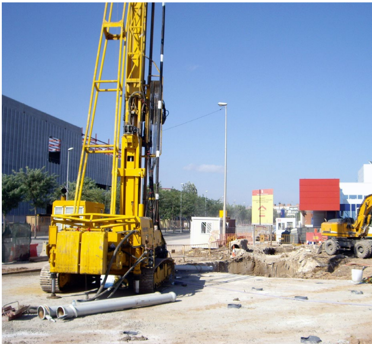
Fig. 33 Details of the PACCHIOSI P1500 ES hydraulic drill rig.
