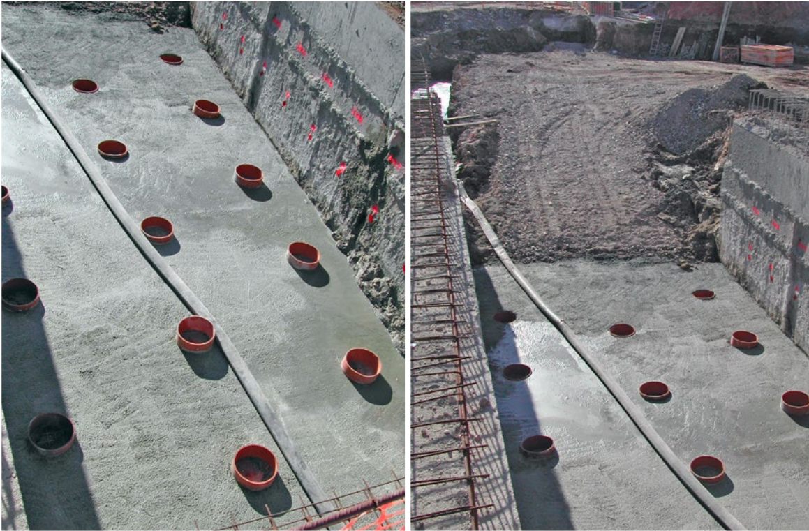
Fig. 15-16. Reinforced concrete slab with preparation of preliminary holes for performance of treatments.
