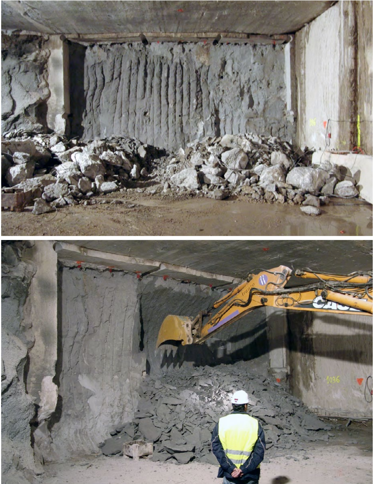
Fig. 13-14. Excavation of the consolidated soil mass with the MEGA JET GROUTING PS3 method.
