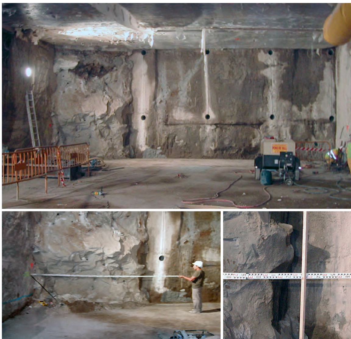
Fig. 10-11-12. Measurement of a closing column between right angle diaphragms.
