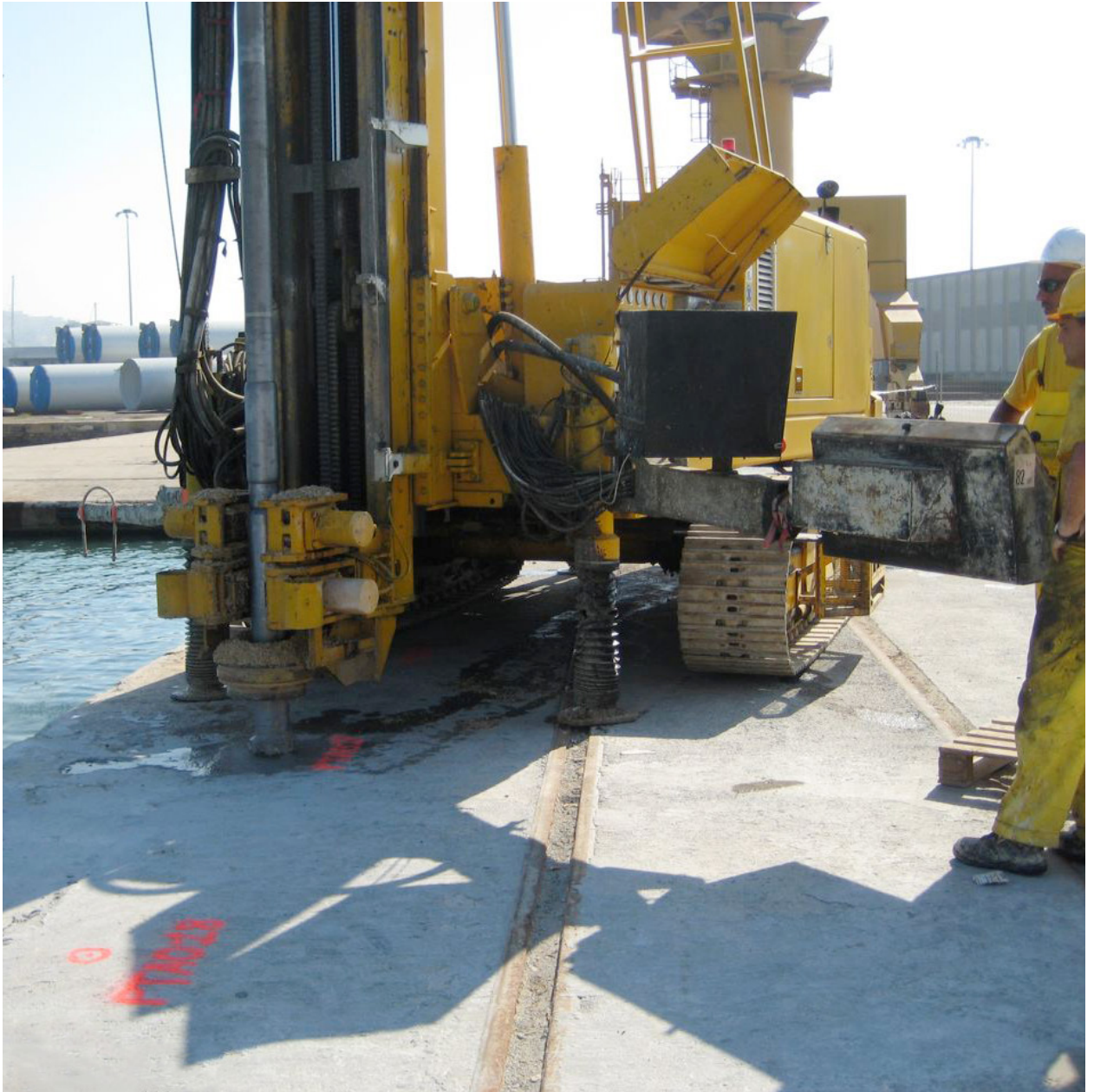
Fig. 5. Phase of drilling through the caissons with DTH hammer
