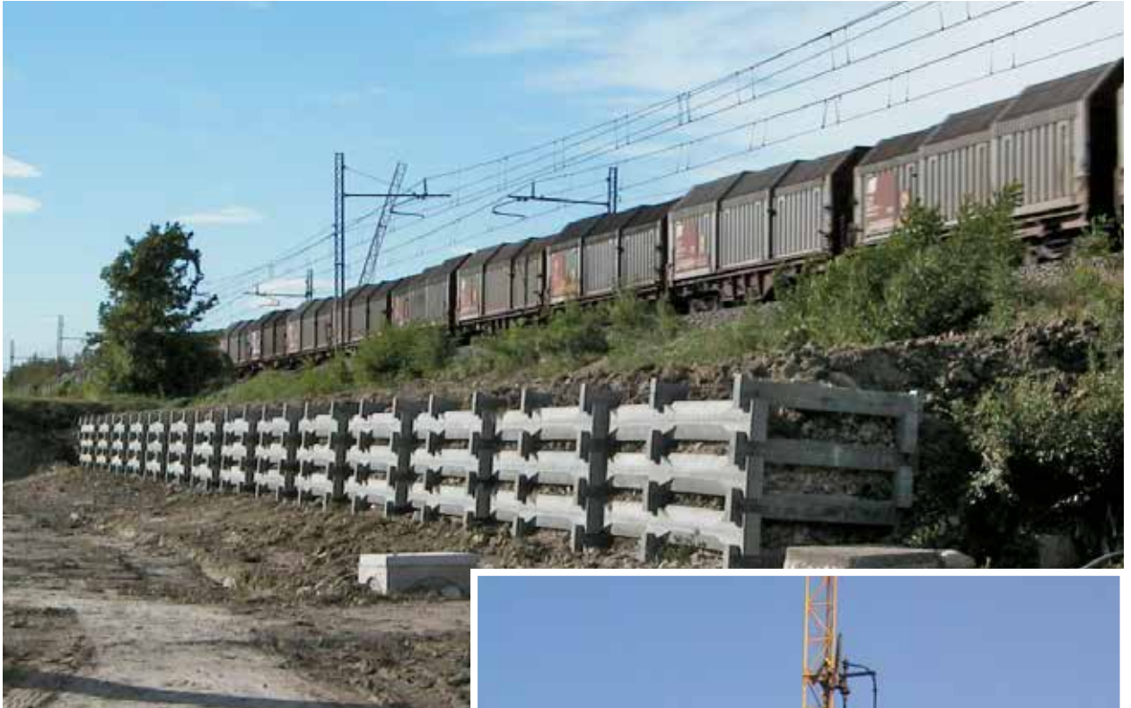
Fig. 6. Prefabricated cellular walls.
