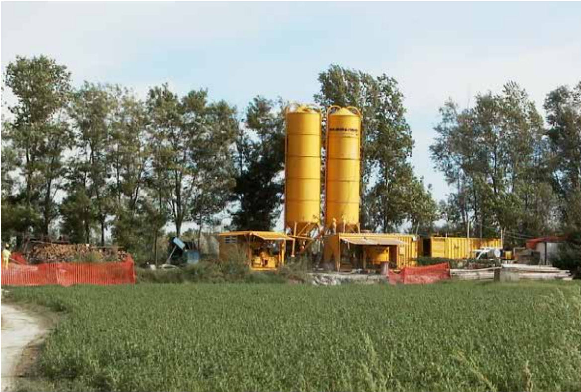
Fig. 8. View of the worksite.
