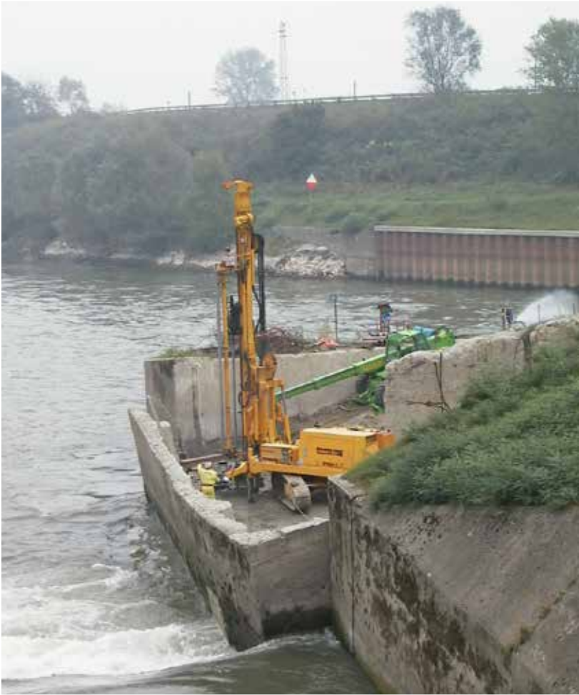
Fig. 4. P 1500 ESCR drill rig for Jet Grouting.
