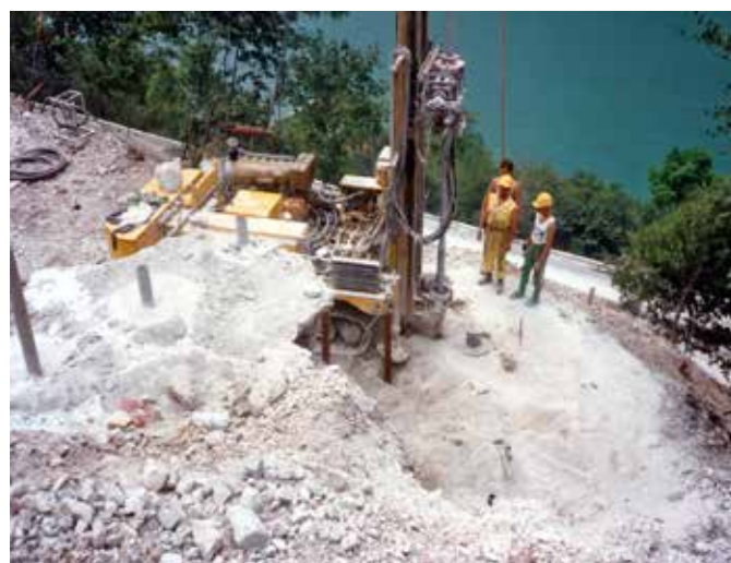
Fig. 4. P 800 drill rig executing the Jet Grouting columns to form the protective collar.
