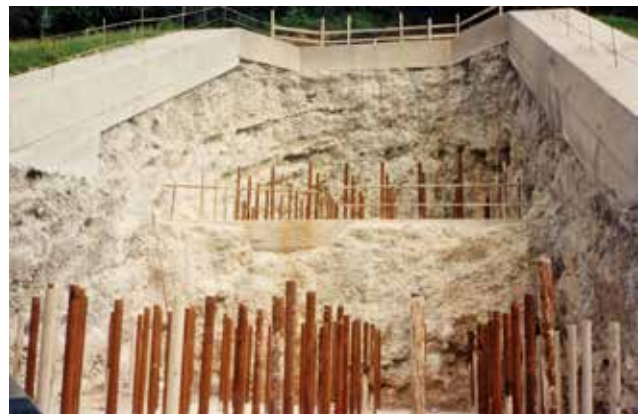
Fig. 12. View of columns' reinforcements.
