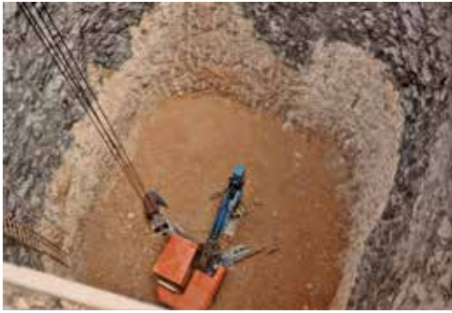
Fig. 9. Excavation of the shaft.
