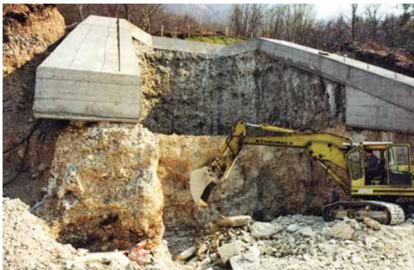
Fig. 6. Excavation for the construction of the foundations.
