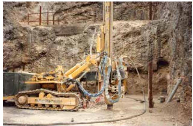
Fig. 11. PRP 105 drill rig during the reperforation of the columns' nucleus.
