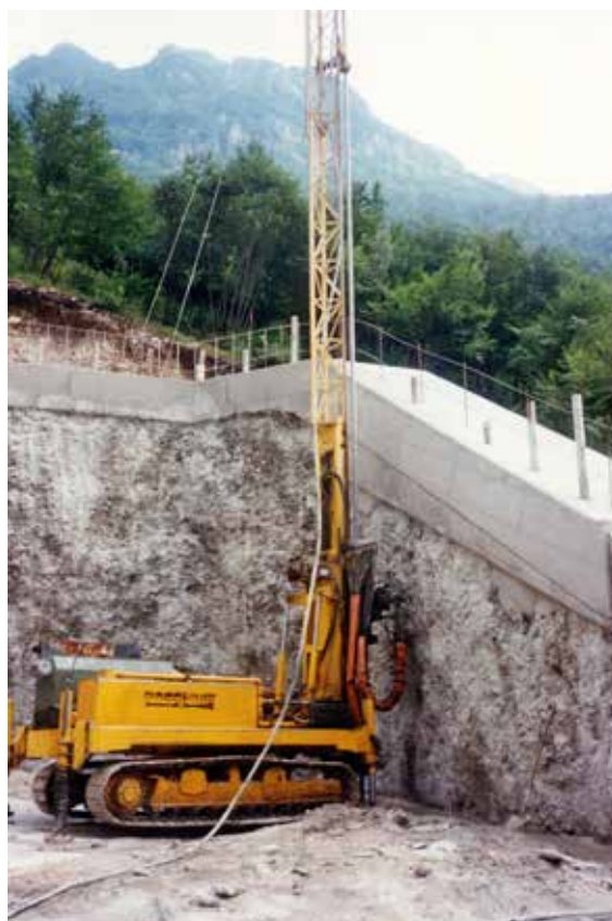
Fig. 8. P 1000 drill rig during the rehalization of Jet Grouting columns.
